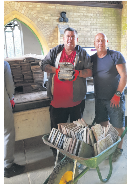
● Unloading of the Victorian tiles
